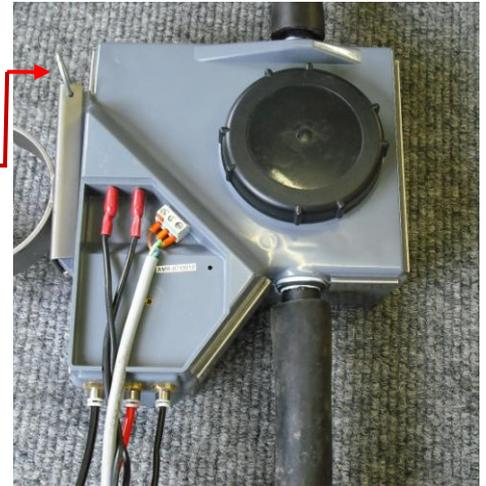
4. Fit the power push on connectors. (either way around). Because the power is low voltage a.c. and isn't polarized
